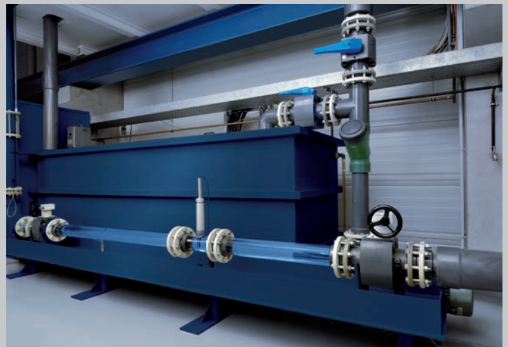
Water calibration installation, nominal values up to DN150
